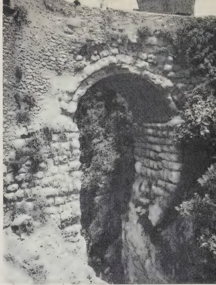
A Roman arch in Italy supports a road still in use
